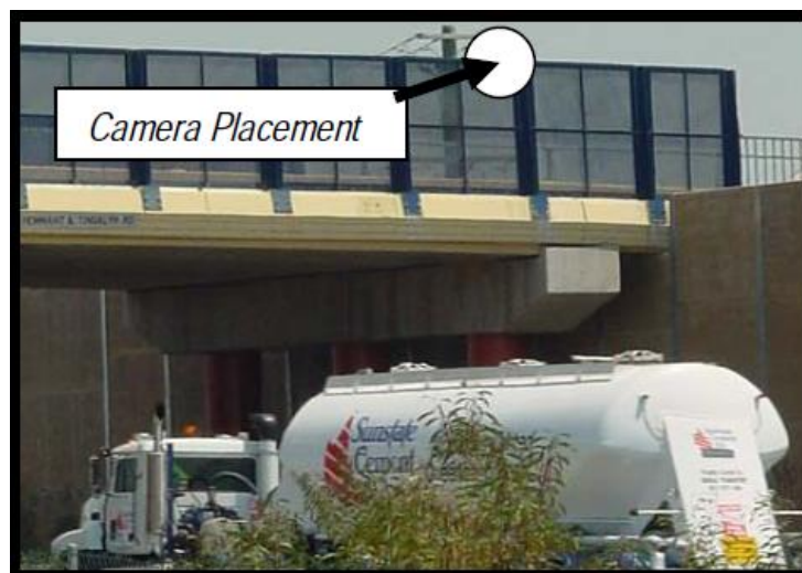
Figure 5 Camera mounted on the overpass (Bunker, 2005)
