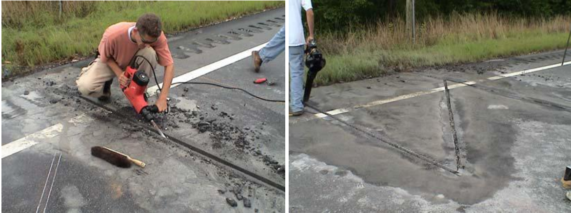
Figure 8 Sensor slots (Timm and Priest, 2005)
