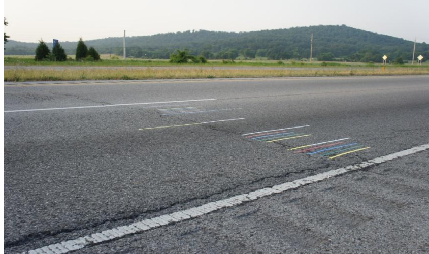
Figure 18 Mark of reference lines in the field
